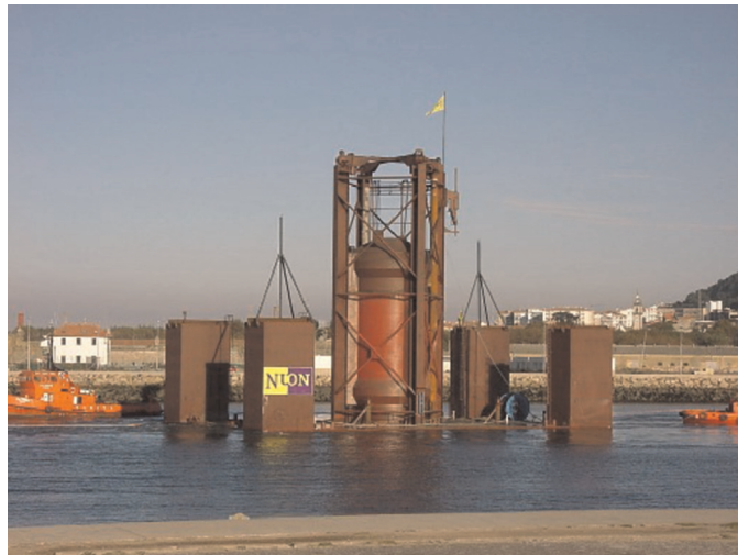
Figure 2. The AWS pilot plant before submersion.
